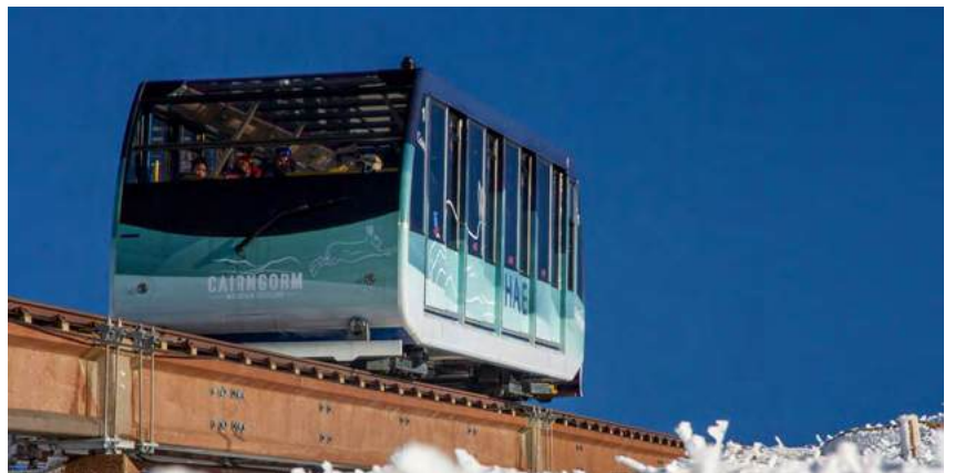
Cairngorm Funicular Railway in operation
